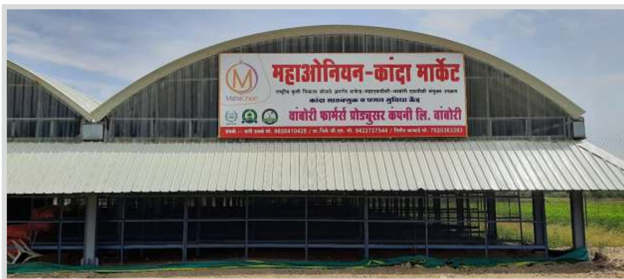
Figure 5.3: Storage System at Vambori FPC
